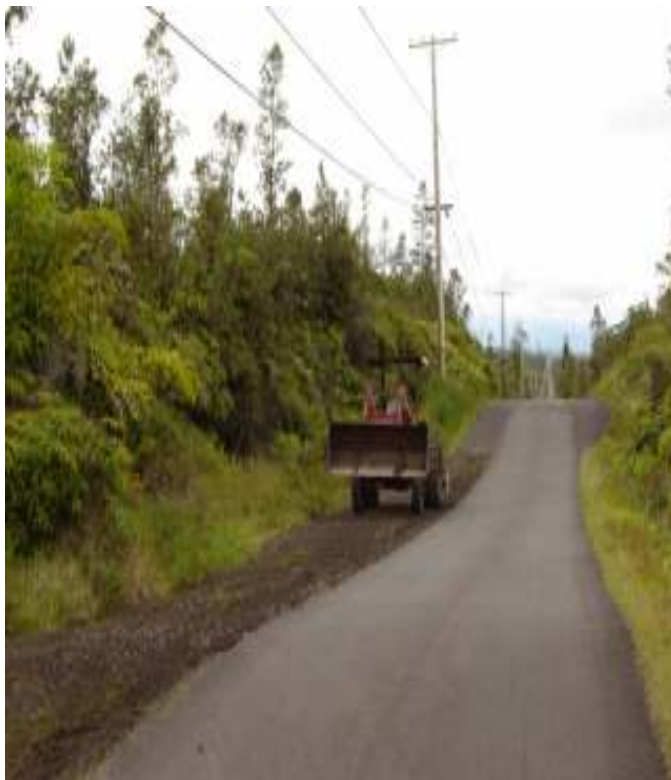
1 RD SHOULDERS BEING MAINTAINED
